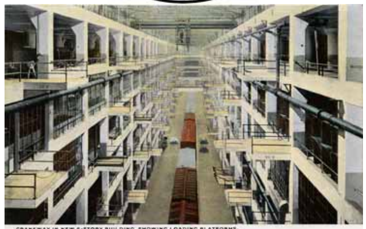
"Craneway in new 6-storey building, showing loading platforms." Postcards showing the Ford plant in 1917.
